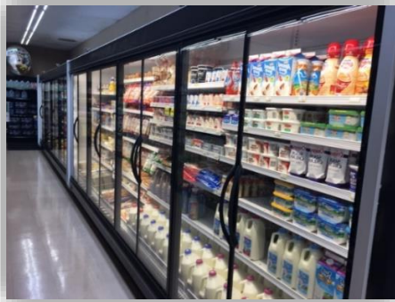
Energy Efficient Refrigeration Cases
