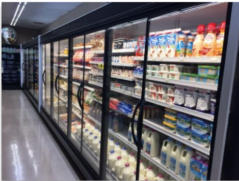
Energy Efficient Refrigeration Cases
